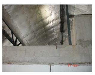
Fixing method illustration when fixing Polynum onto existing metal trusses for new or exiting structure:
